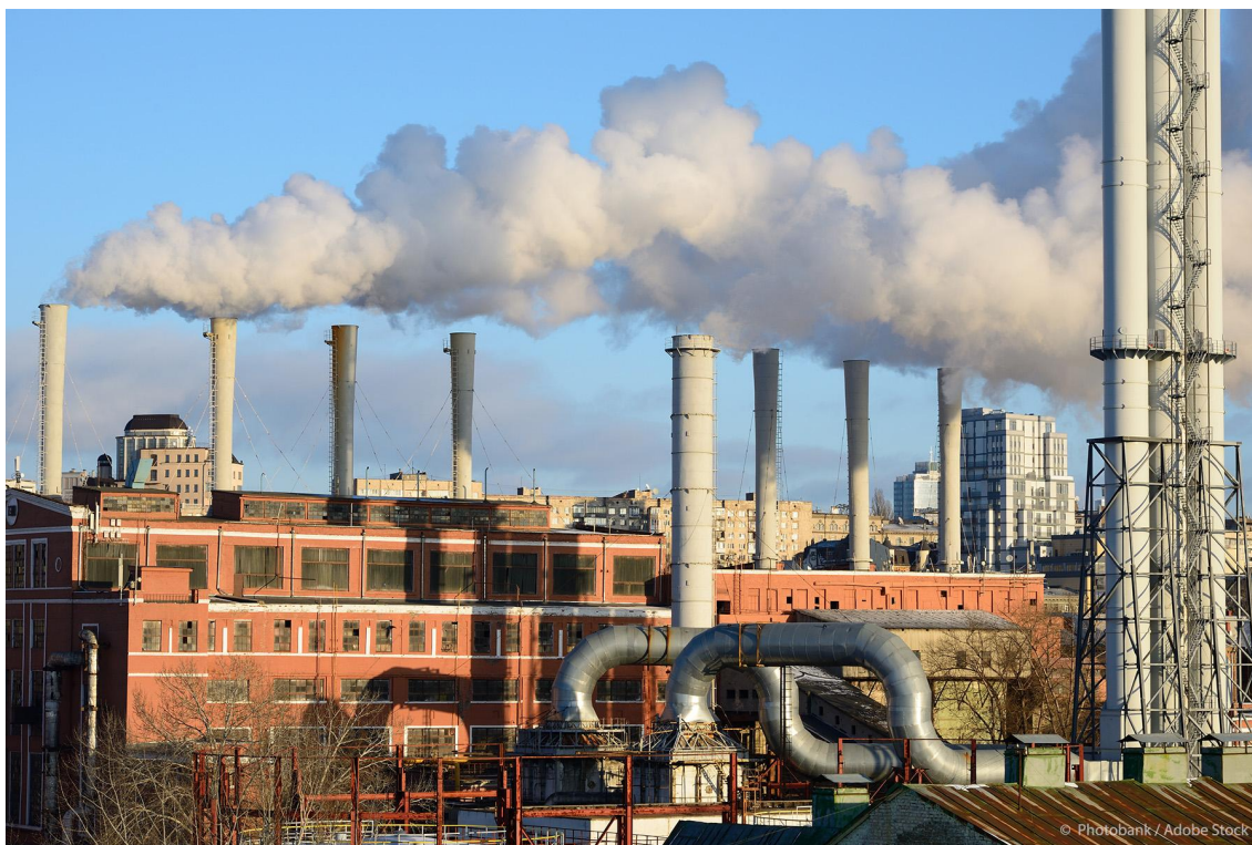
Heat station in the city
